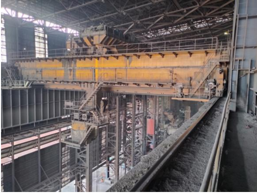
Monitoring system at a crane
