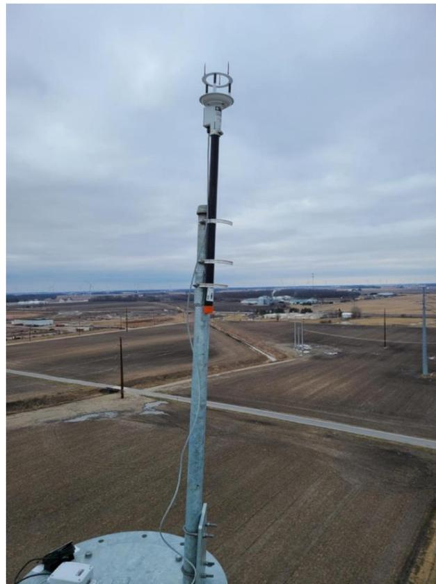
Figure 4: An installed Resensys wireless Anemometer SenSpot™ on top of a utility tower
